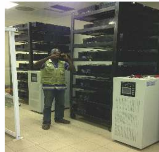
120KVA (60Kva each) Inverter Installation National Stadium, Abuja
