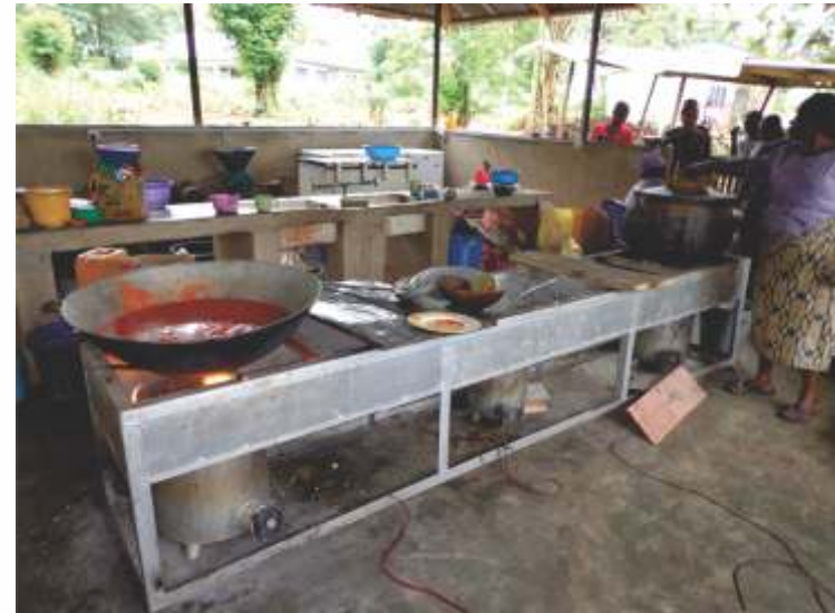
Quintas 12", 10" and 8" Biomass stove array at Arch Bishop Vining College, Akure
